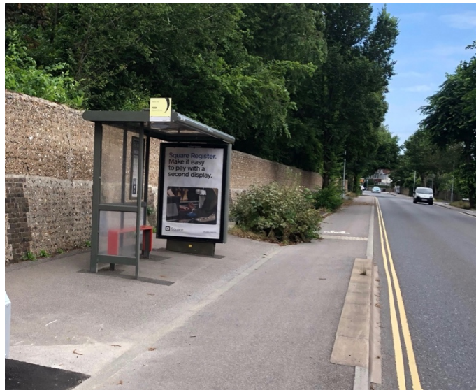
An existing bus boarder in Old Shoreham Road showing the poorly marked cycle lane between the bus stop and road. It has no signs instructing cyclists to slow or give way. This part of Old Shoreham Road has an hourly bus service. The stops in Preston Road and London Road are much busier with very frequent bus services.
